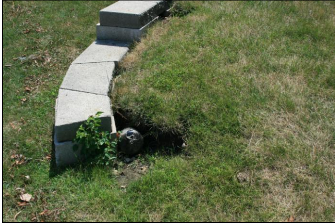
Stormwater runoff has eroded the land around this retaining wall. Photo courtesy of Beth Corrigan
