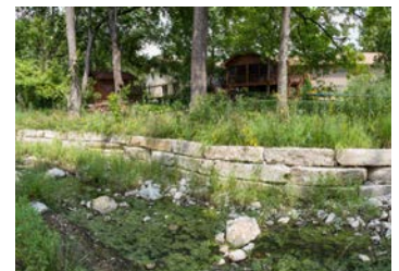
► Example of natural structural retaining wall
