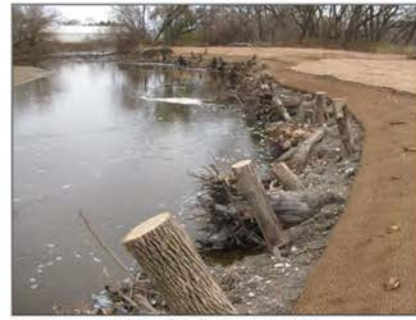
Image: post-construction crib-wall, pre, pre-vegetation.
