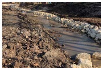
► Example of toe of slope construction in progress with a floodplain bench
