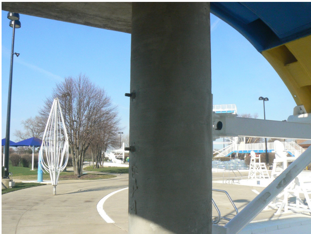
Slide attachment to northwest column
