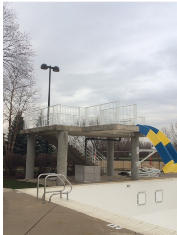
North Elevation of 3m Diving Platform
