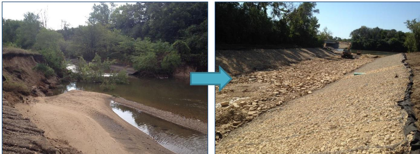
BLA also provided construction engineering services. During the work, a heavy rain event eroded much of the already completed side slopes at the Rock River Outfall and a portion of the existing concrete spillway broke away. Side slopes needed to be regraded while the concrete spillway limits were revised because of the storm damage.
