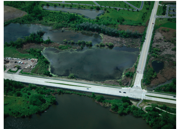
Civiltech's Mateen Baig provided Construction Inspection on IDOT's US 6 (159th St.) Reconstruction project .
