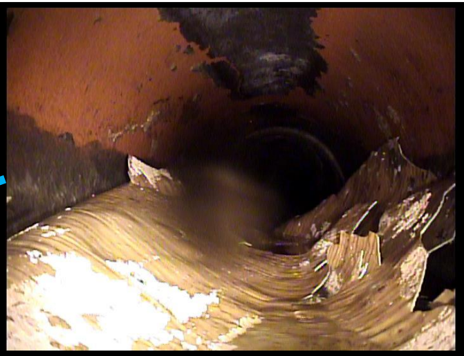
Previous 2004 repairs of epoxy resin liner of manholes in pipe
