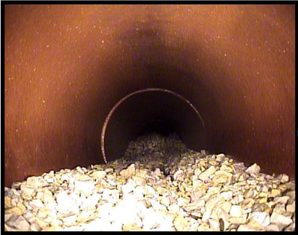
Stone Debris found in pipe
