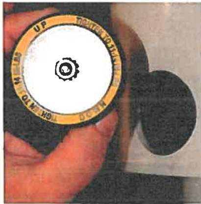
Figure 17 Placing rubber plug over access hole
