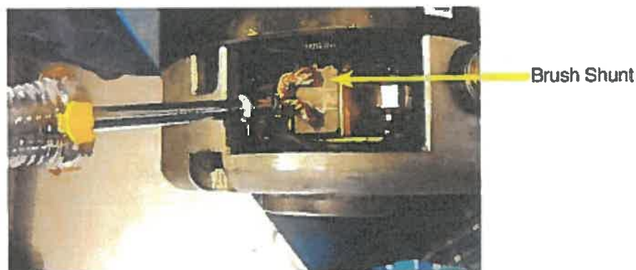
Figure 22 Removing Brush Shunt Bolt
