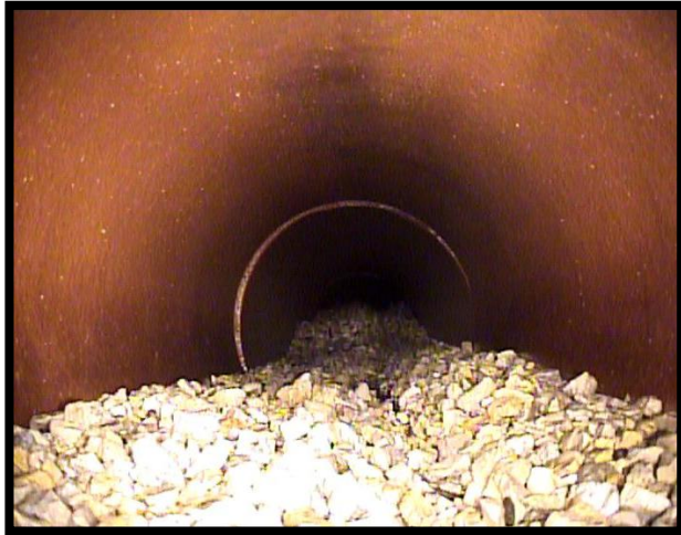
Stone Debris found in pipe
