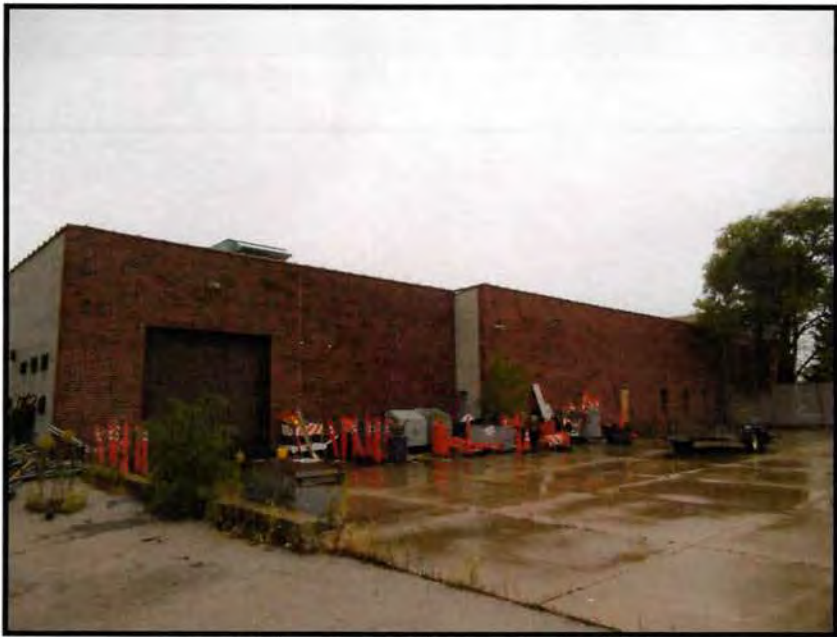
North Elevation of the Subject Property
