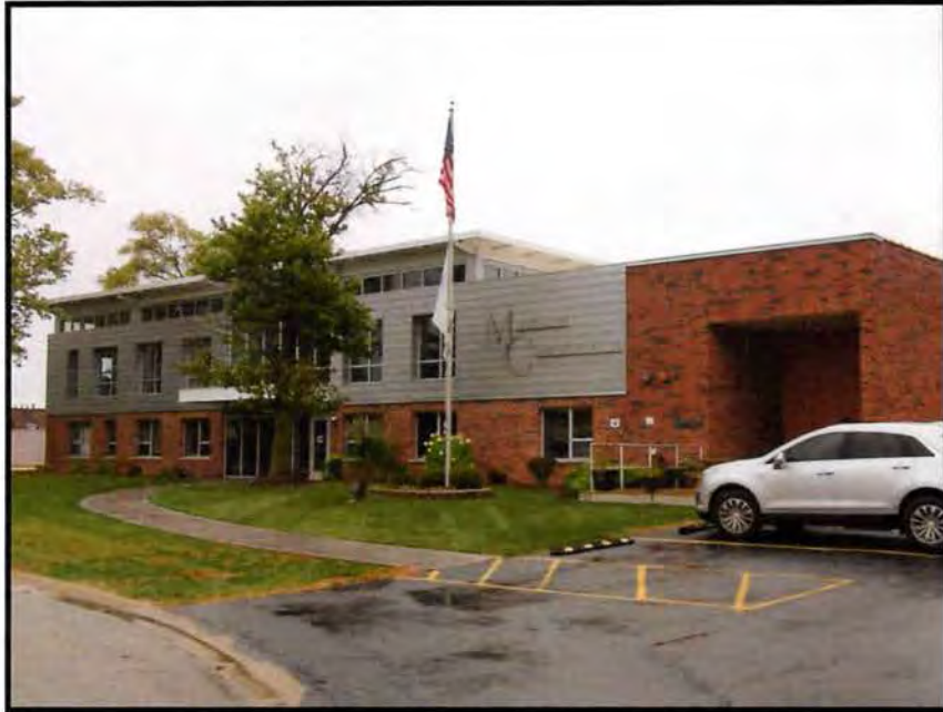
West Elevation of the Subject Property
