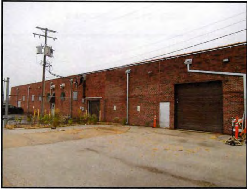
South Elevation of the Subject Property
