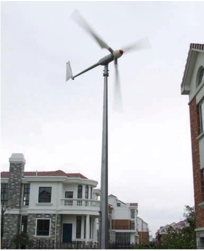
Figure 5: Example of a freestanding MINIWECS monopole turbine
