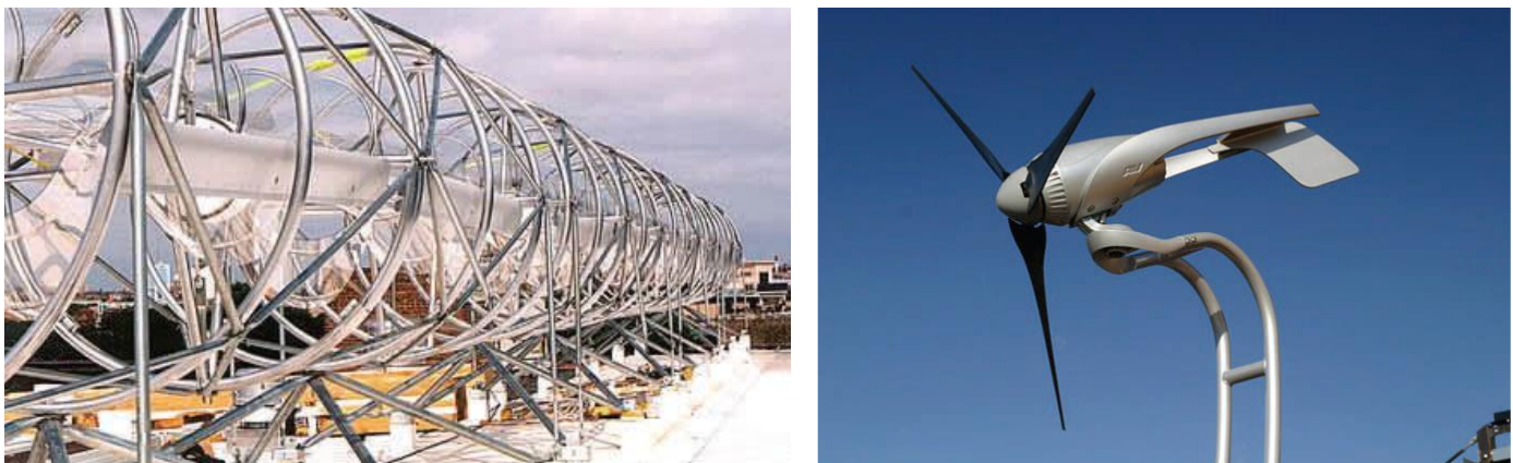
Figure 4: Examples of MINIWECS roof-mounted turbines oriented horizontally and vertically
