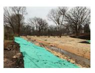
Example of turf seeded area with netless blanket to the top of slope
