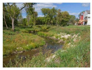
► Bio-engineered bank stabilizations in floodway
