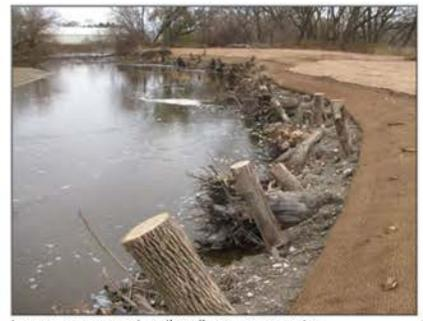
Image: post-construction crib-wall, pre, pre-vegetation.
