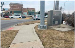
**Figure 2. SE Corner.** Highlighting no pedestrian accommodations or crosswalk.
