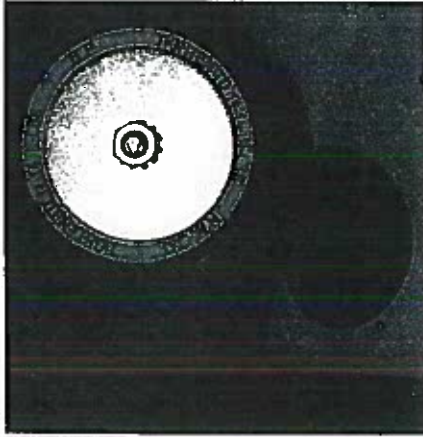
Figure 17 Placing rubber plug over access hole
