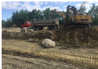
Construction of Veteran's Memorial Peninsula
