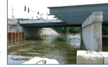
BLA provided both inspection and design services for the reconstruction of the IL 64 Bridge over the Des Plaines River. BLA provided services from the TS&L phase to the final plans and specifications. BLA designed a three-span, sevenlane, steel beam bridge to be constructed in stages while maintaining traffic in both directions. Bridge work also
