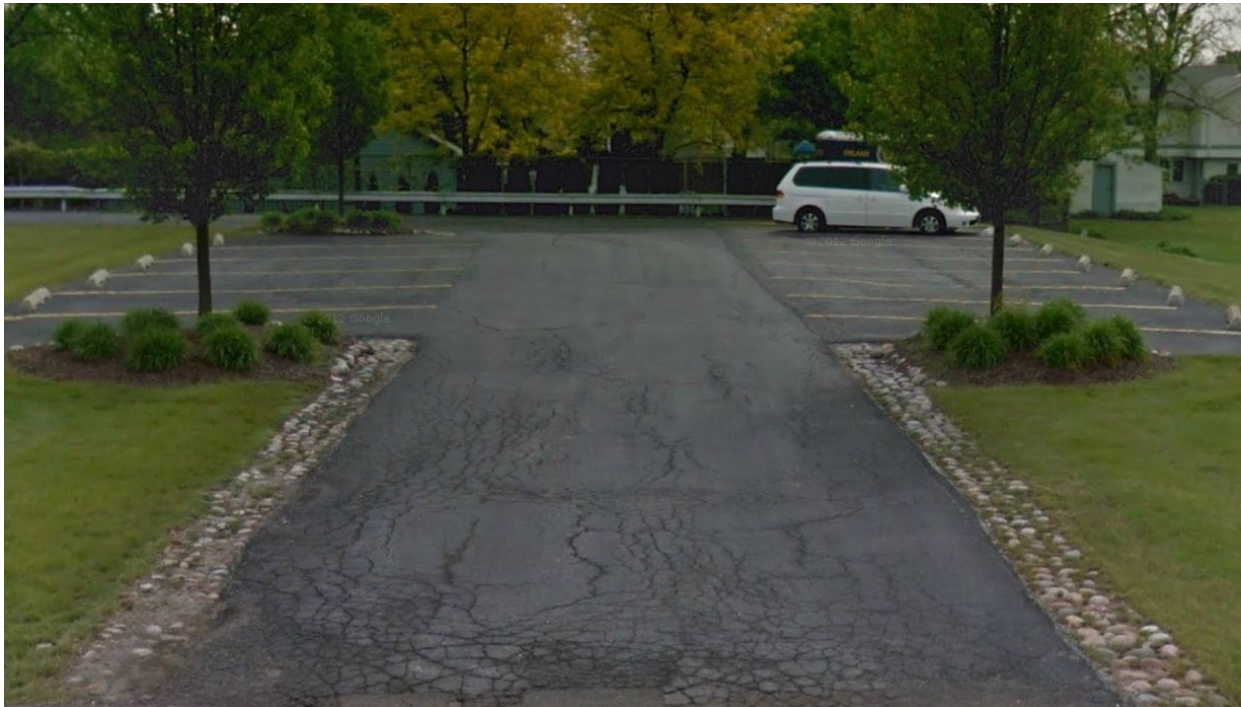
Figure 1. Example of a Village parking lot rehabilitation candidate.
