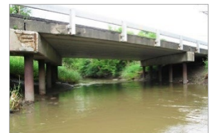
Existing bridge – superstructure replacement is proposed.
