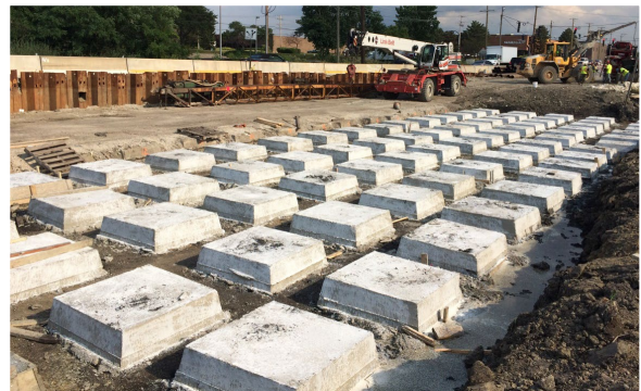
A main component of the project is the dryland bridge design and potential separate contract.
