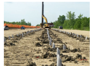
Example construction of wick drains.
