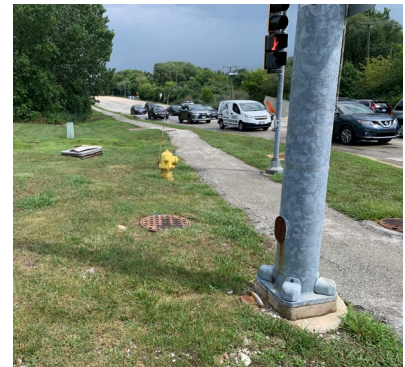
Our field investigation indicates the existing water main and fire hydrants (shown in blue line) may be in conflict with the roadway, dryland bridge, and/or storm sewer requiring relocation.
