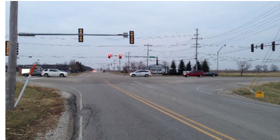
US 34 and Eldamain Road traffic signal equipment was modernized for the added turn lanes.
