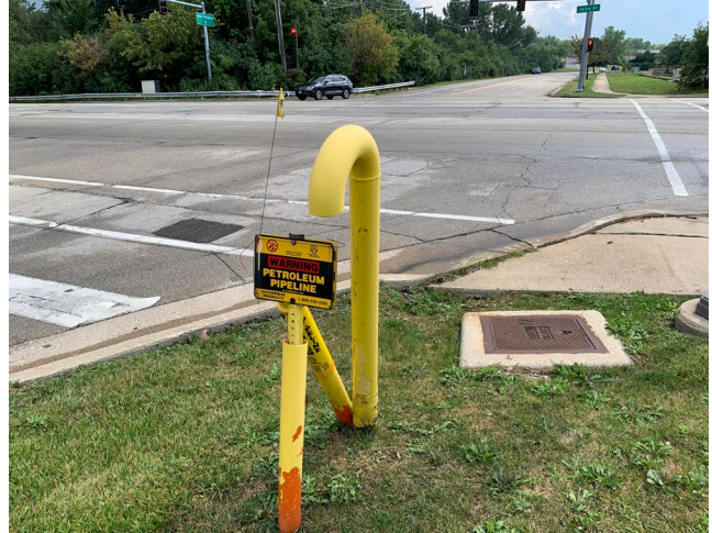
A focus on coordination with private Utilities will assist in preventing delays during construction.
