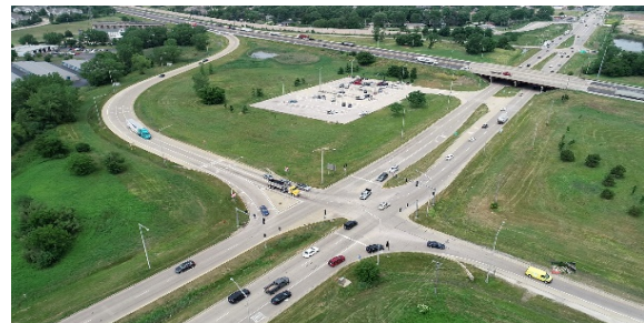
US 30 at I-55 included two signalized intersections with street lighting.
