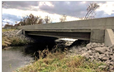
Single-span PPC I-Beam bridge replaced existing triple 60-inch CMP culverts.
