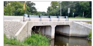
Completed dual-cell box culvert.
