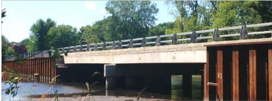
Completed Hill Road Bridge – walls were provided to avoid floodplain fill.
