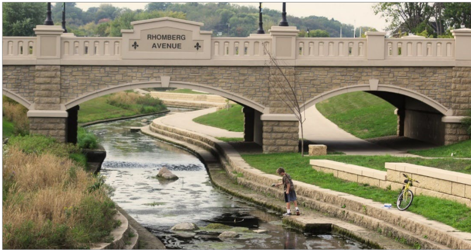
Stunning arch bridge over the Bee Branch River.
