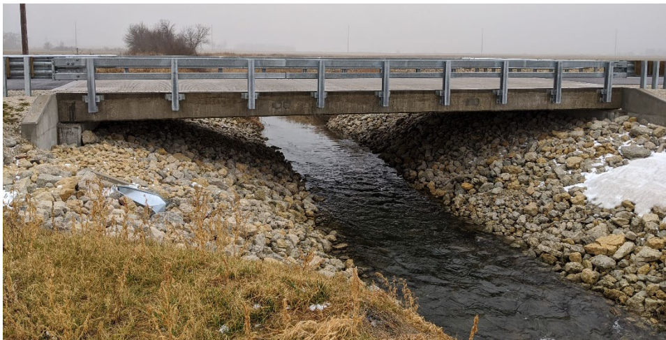
Completed Base Line Road Bridge over Coon Creek; a creative design avoided ROW or temporary easement acquisitions.
