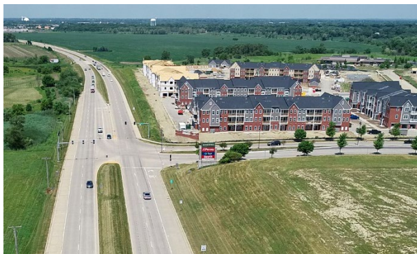
One of four Signalized Intersection that were reconstructed and modernized.
