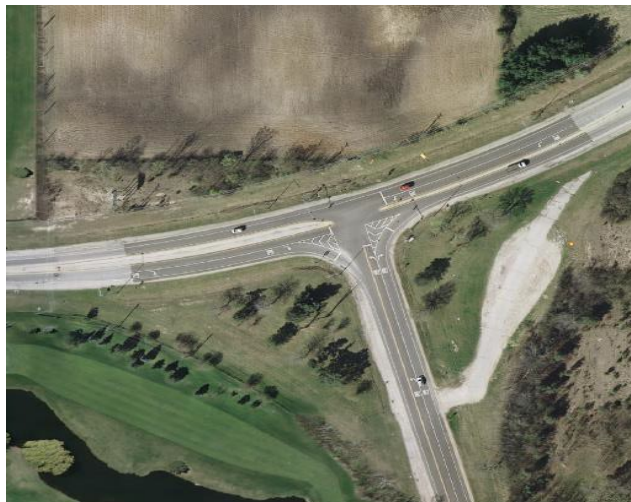
IL 47 at IL 176 East – existing T-intersection with no right-turn bypass lane.
