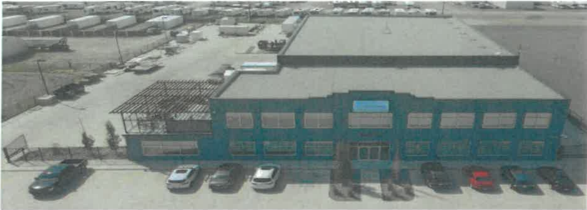
Flowpoint Headquarters, Morinville, Canada.
