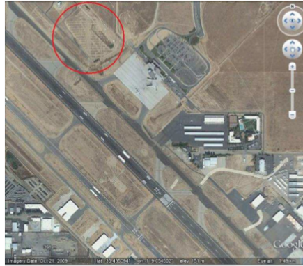
Figure 7: Bakersfield Airport showing location of solar array
