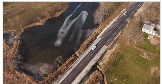
Aerial view of culvert improvements
