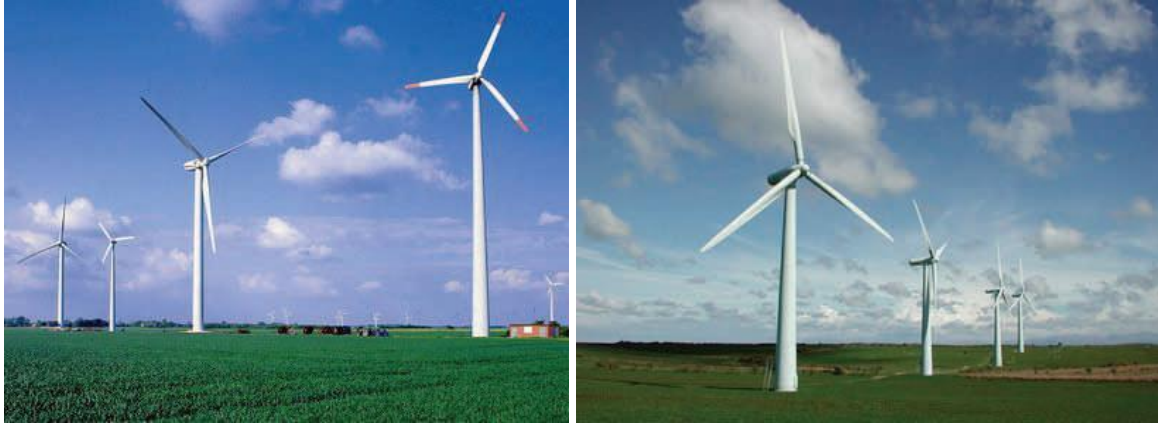
Figure 9: Examples of a UWECS solar farms
