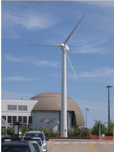
Figure 8: Example of a SWECS with horizontal axis rotator blades
