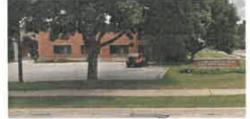
Public Works Facility Village of Downers Grove
