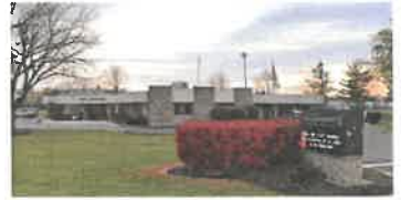
Police Department Renovation Village of Shorewood
