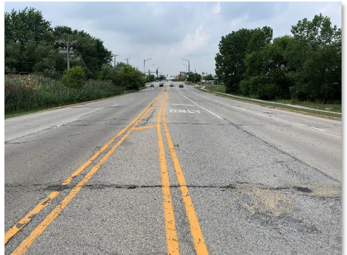
Existing dryland bridge on 143 rd St., looking West towards intersection
