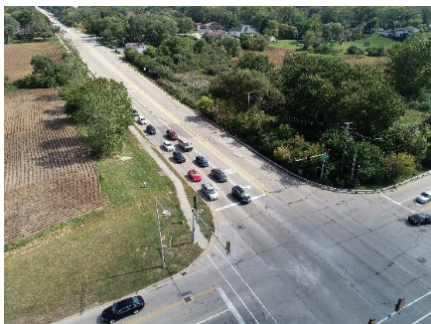
Looking West at the Dry Land Bridge
