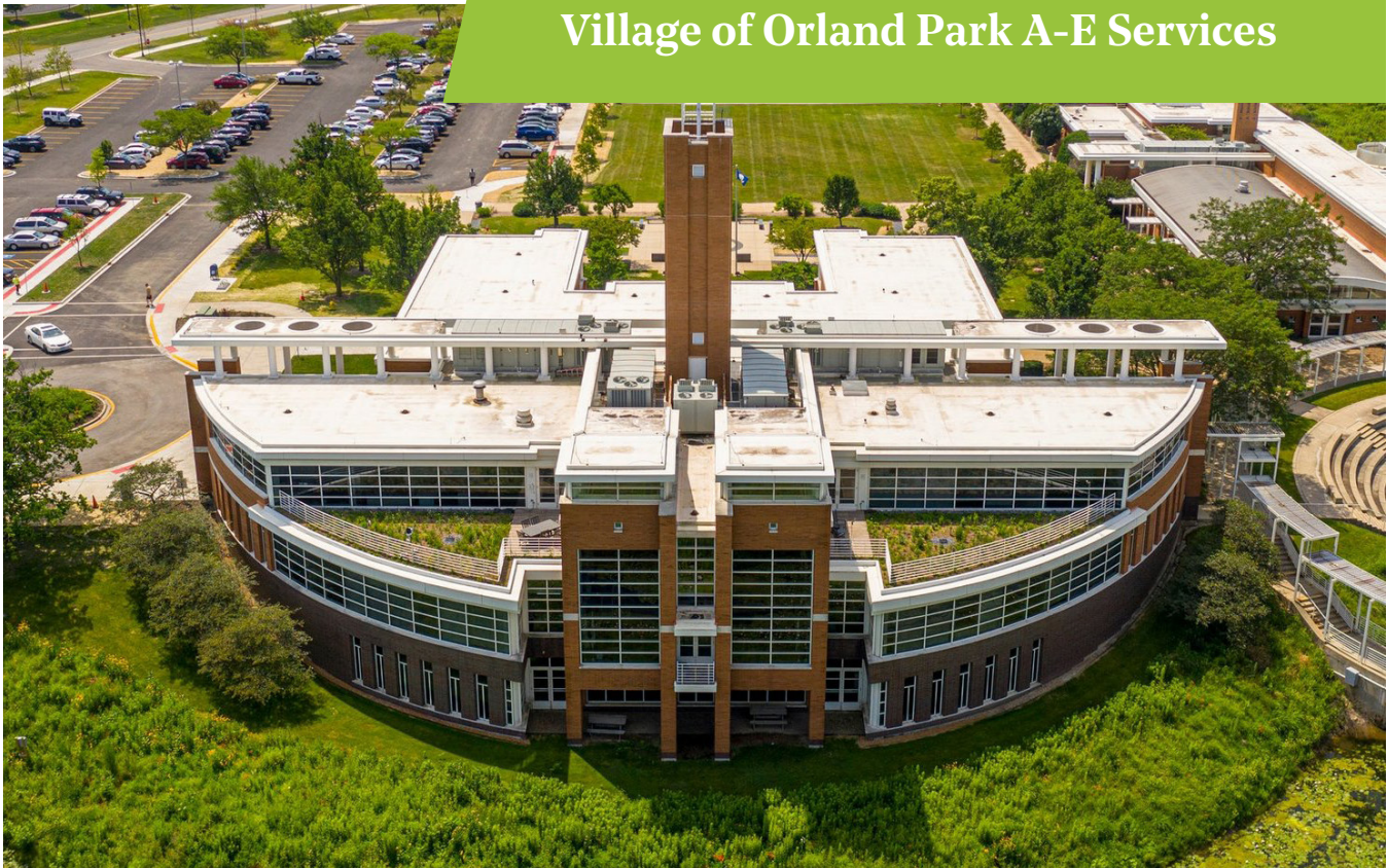
Village Hall – photo credit: https://ecogardens.com/orland-park-green-roof
