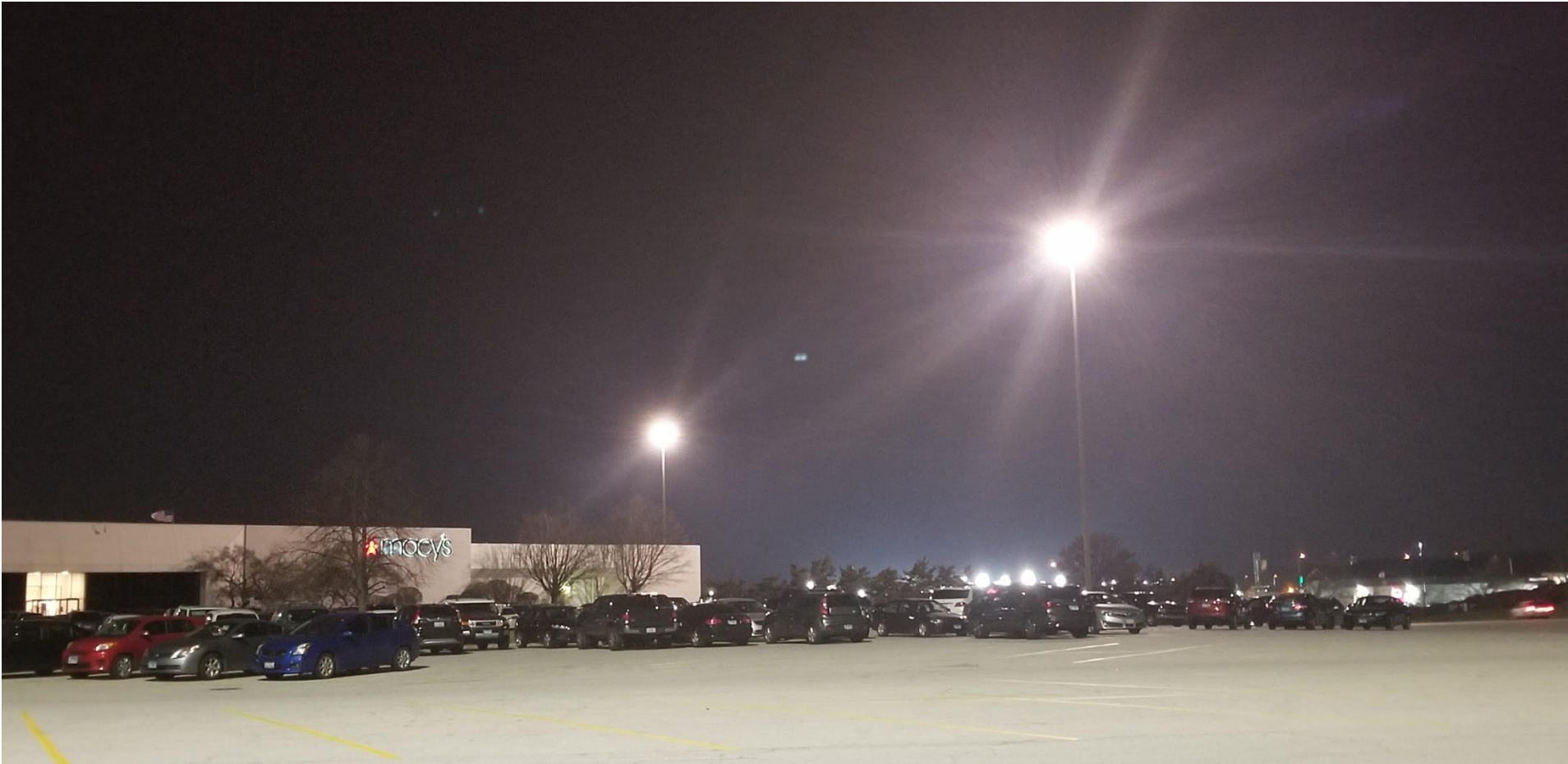
Subject Light Poles (Photo Taken Facing West)
