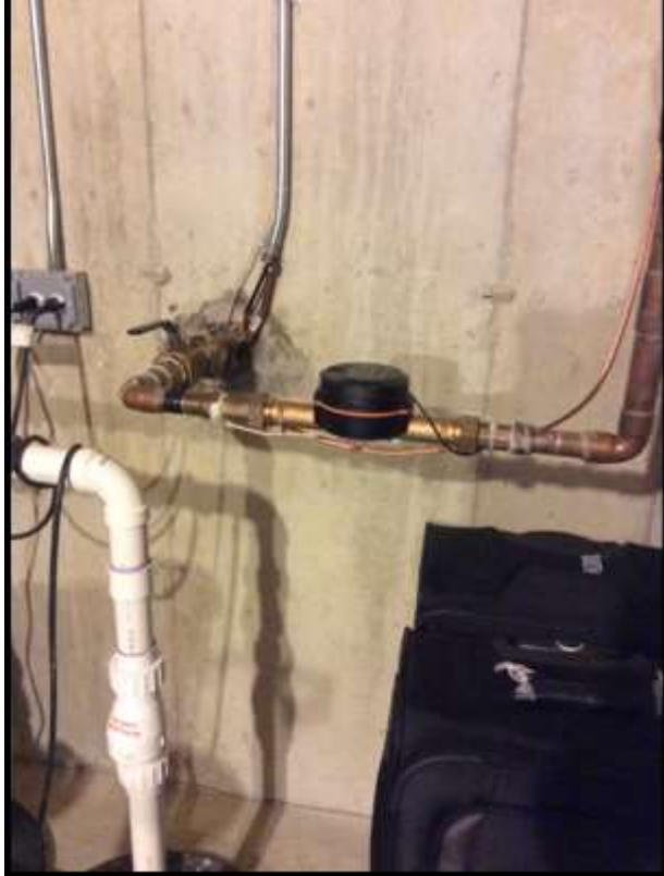
Completed Installation Photo
