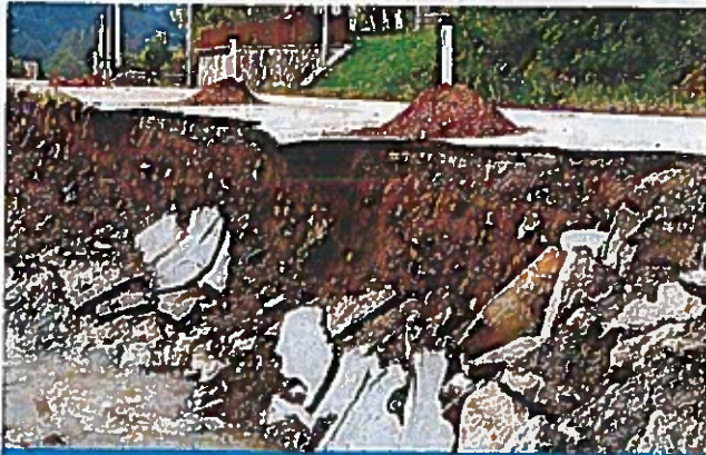
LANDSLIDE MONITORING AND DETECTION
