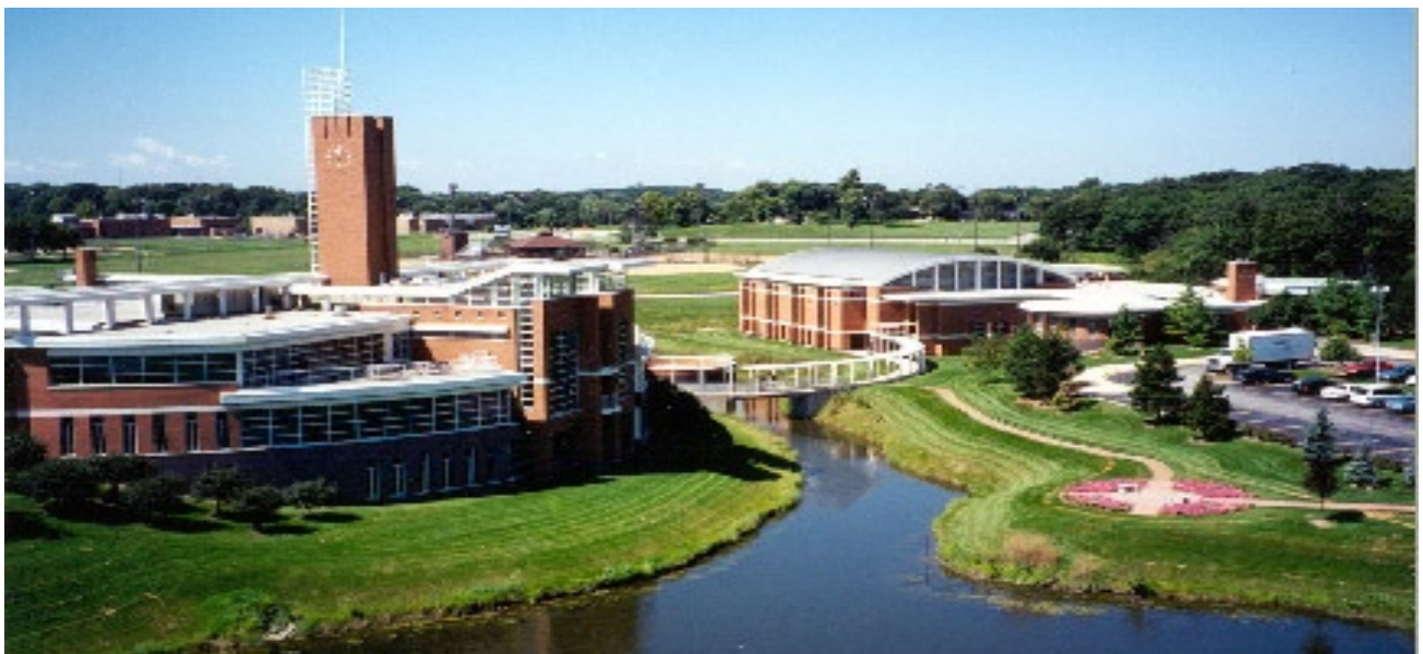
Civic uses like the Metra Station, Library and Village Hall are the focal points of the Village Center District
