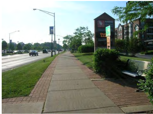
Examples of sidewalks and parkway treatments along suburban arterials.
