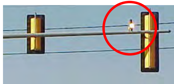
Transit signal priority beacon (top) and activated by a vehicle (bottom). Source: Village of Mount Prospect.
