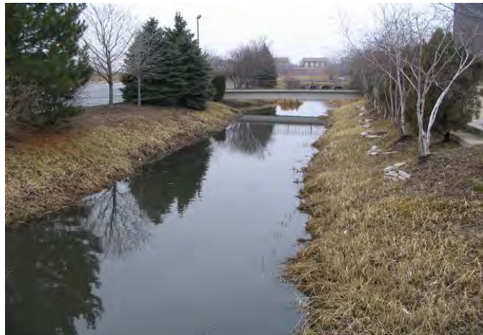
Open stormwater drainage integrated with landscaping near in the South-Center section near 156 th Street
