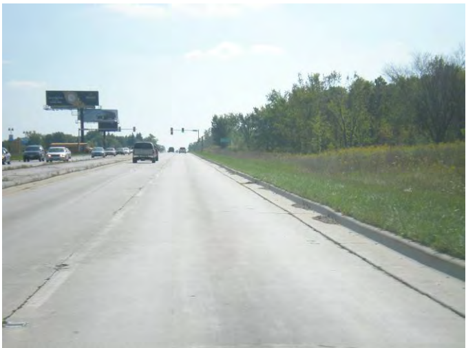
La Grange Road in the south section along the Orland Grassland Forest Preserve
