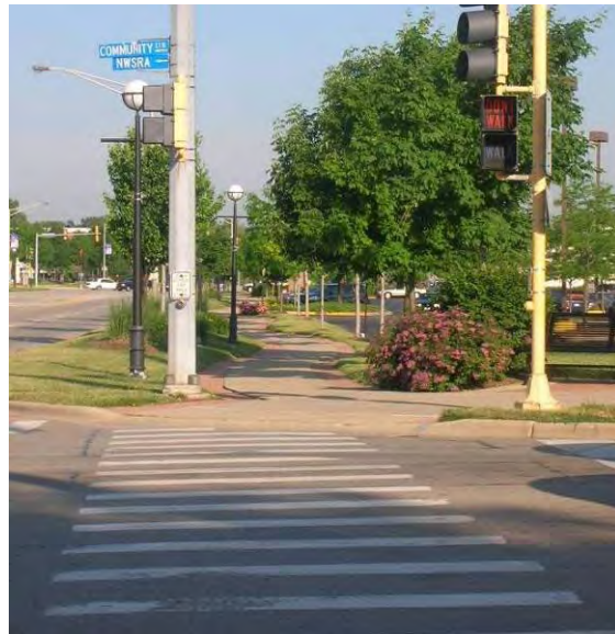
Pedestrian crossing with continental style pavement marking.
