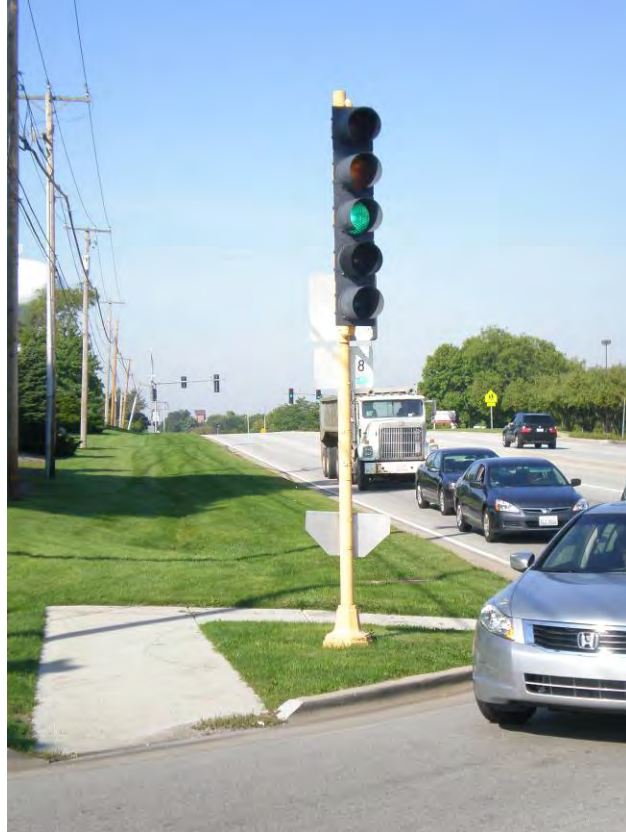
Wide parkways are frequent in the North section along La Grange Road but sidewalks are lacking in some areas.
