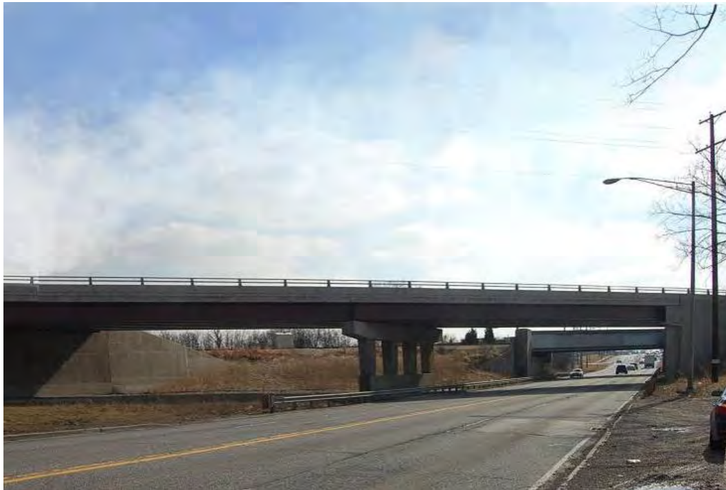
Existing Southwest Highway Bridge
