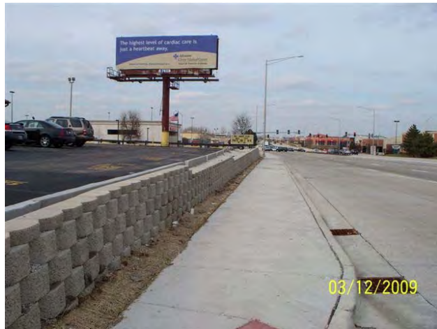
Retaining wall along La Grange Road near 159 th Street. This would be the standard under the IDOT proposed plans.
