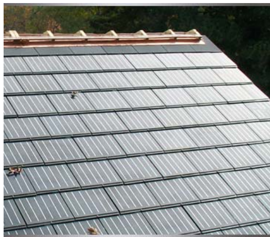
Solar roofs, such as the one at left, can be retro-fitted on historic buildings such that the SES appear as if they were asphalt shingles. Section 6-209 Old Orland Historic District permits asphalt shingles as an appropriate roofing materials in the historic district.
