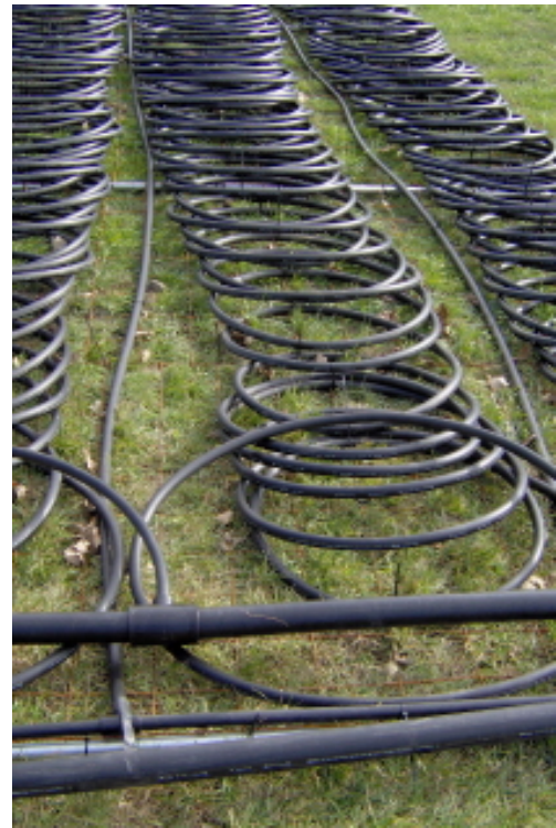
Left: Renderings that show residential and non-residential applications of hydrothermal heat pump systems using detention ponds. Above: Pond loop coils prior to being submerged into a pond. Orland Park has many residential and non-residential detention ponds that can be used as heat sources and sinks for improved energy efficiency.
