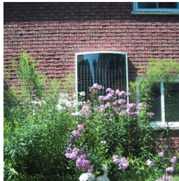
Above: Solar air heating systems attached to the façades of residential buildings. Light screening is recommended when facing public right-of-ways. Wall-mounted SAH units should face south for greatest exposure. Below: PV and SAH on a multi-family, mixed-use building.
