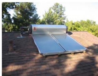
SLH systems should be flat on rooftops or walls. Systems with attached tanks (left) should be aerodynamic and light-weight. Upright SLH, such as the one at right, is prohibited
