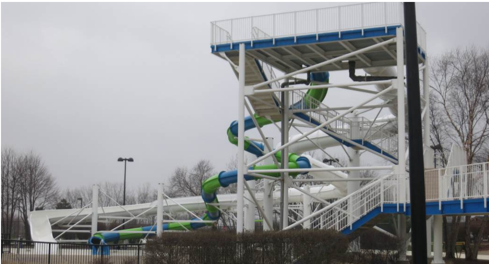
Photo No. 2 – Tall Slide to be investigated.
