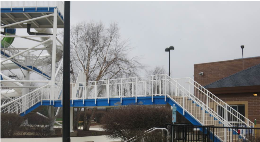
Photo No. 3 - Cross-walkway system to be investigated.
