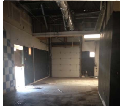
3 Existing building interior
