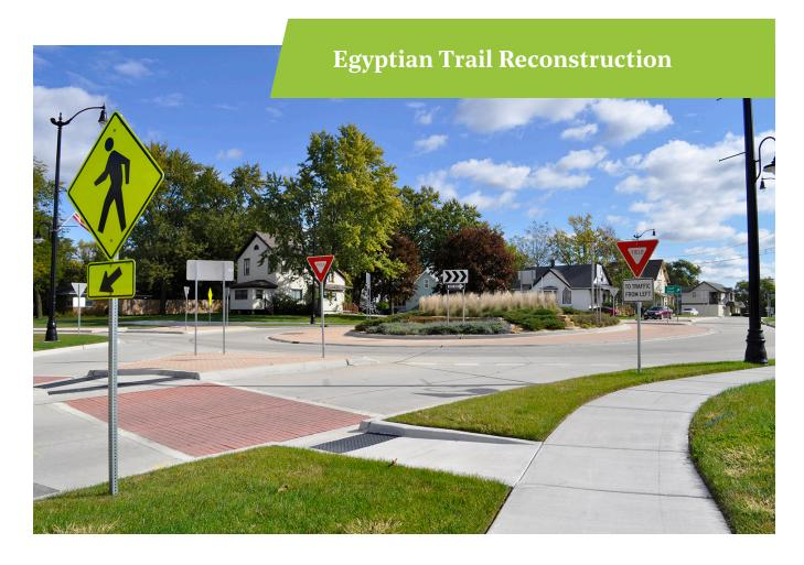
Phase I, Phase II, and Phase III engineering services for the reconstruction of approximately 0.7 miles of the existing Egyptian Trail, which consists of turning a 2-lane rural cross section into a 3-lane urban cross section roadway.
