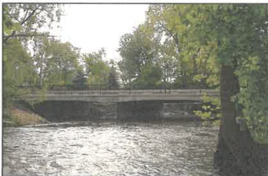
Hillside Road Bridge—Naperville, IL
