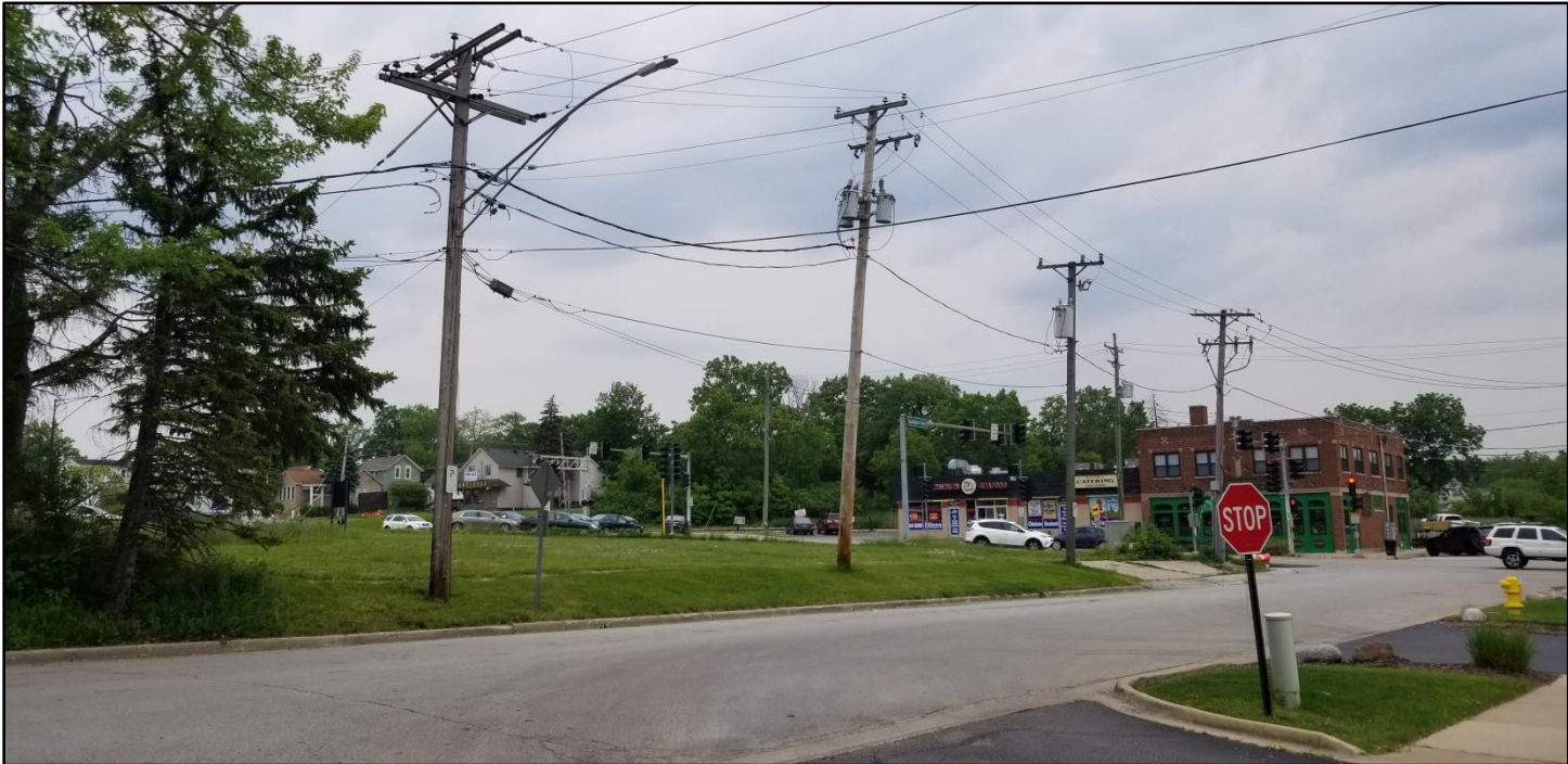
Graphic F: Photo of Existing Overhead Utility Lines on the West Side of the Site
