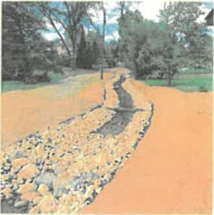
St. Joseph Creek design/build project for Downers Grove included native vegetation slope with rip rap toe.
