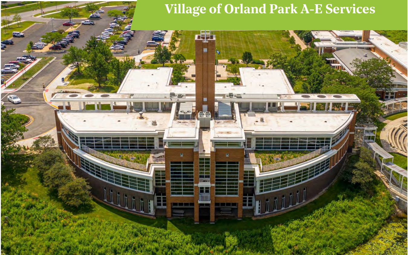
Village Hall – photo credit: https://ecogardens.com/orland-park-green-roof
