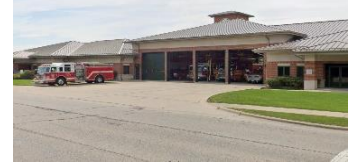
Central Fire Station Deerfield, IL
