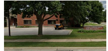
Public Works Facility Village of Downers Grove
