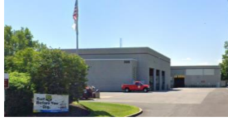
Public Works Facility Village of Lake Zurich
