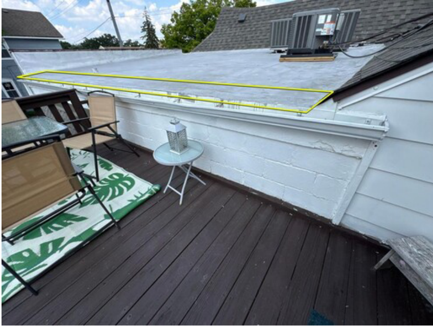
Re-flash roof membrane at gutter edge
