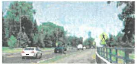
McHenry County DOT - Walkup Rd. Path
