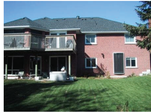
Above: Solar air heating systems attached to the façades of residential buildings. Light screening is recommended when facing public right-of-ways. Wall-mounted SAH units should face south for greatest exposure. Below: PV and SAH on a multi-family, mixed-use building.
