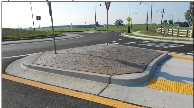
Colored and stamped concrete in the splitter island at Wadsworth Road
