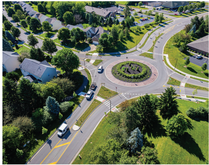
Snider Road and Thornberry Court roundabout.
