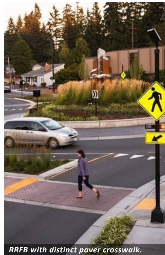
Pedestrian-Actuated Warning Beacon.
