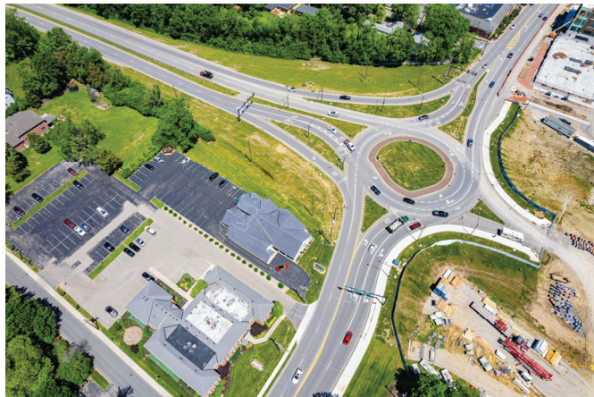
The multi-lane roundabout replaced a separated grade interchange at US 22 and SR 126 and opened in August 2021.
