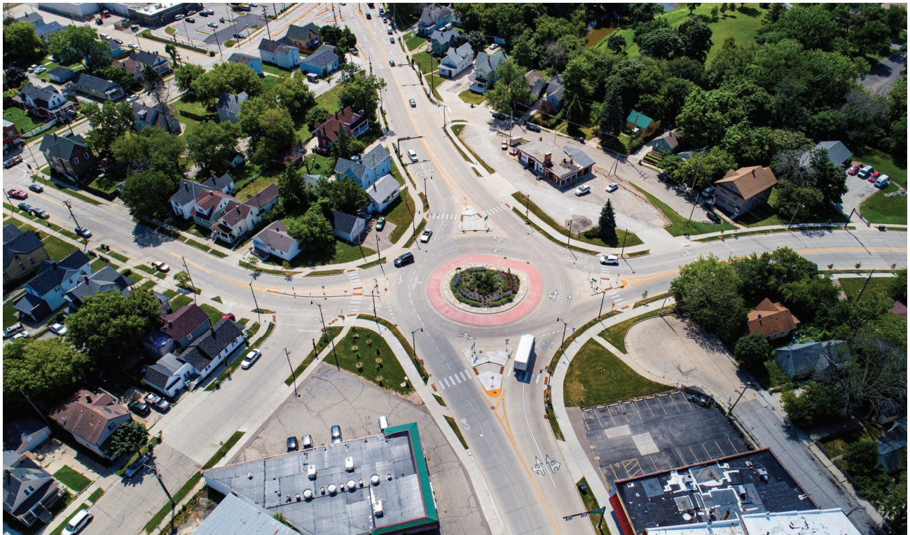
The completed roundabout converted the five-legged intersection into 4 legs and cul-de-sac'd one side road.
