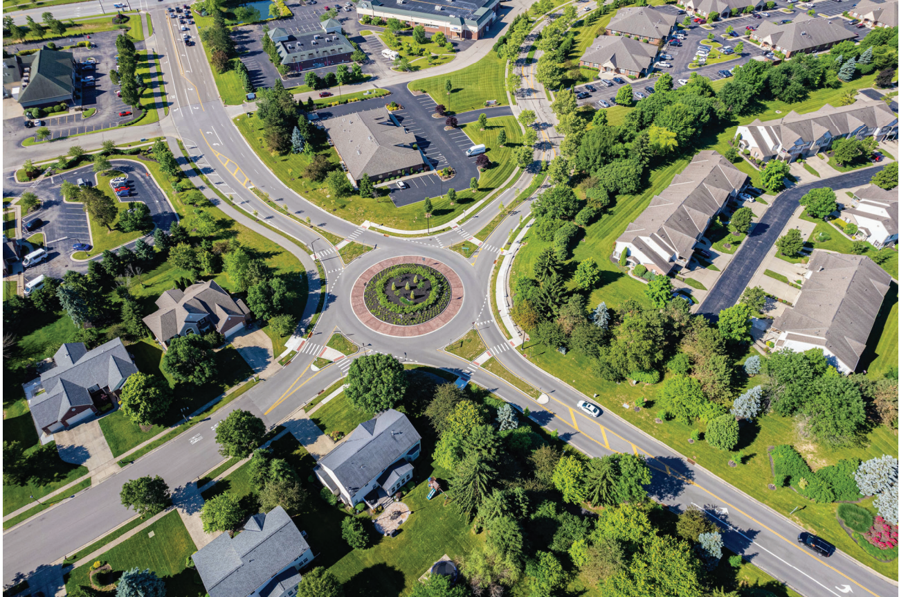
Completed roundabout at Snider Road and Thornberry Court avoided impacts to residential properties.
