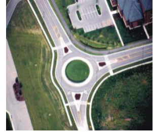
Aerial view of Navajo Drive roundabout.
