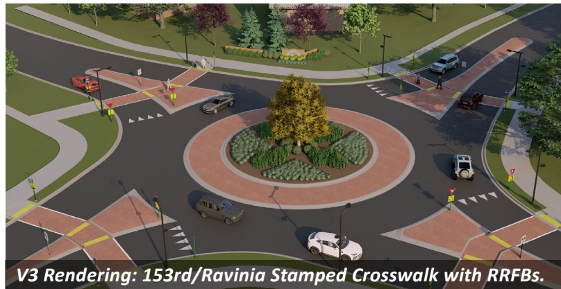
Recently designed roundabout by Strand incorporating RRFBs.
