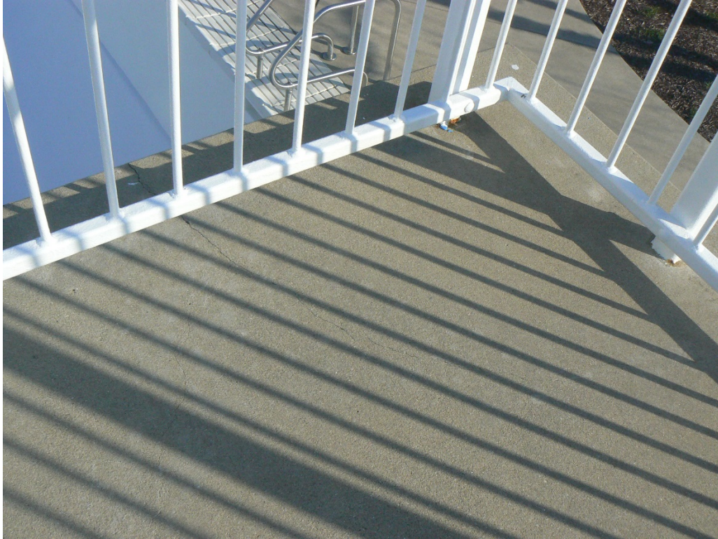
Crack E over top of northeast column
