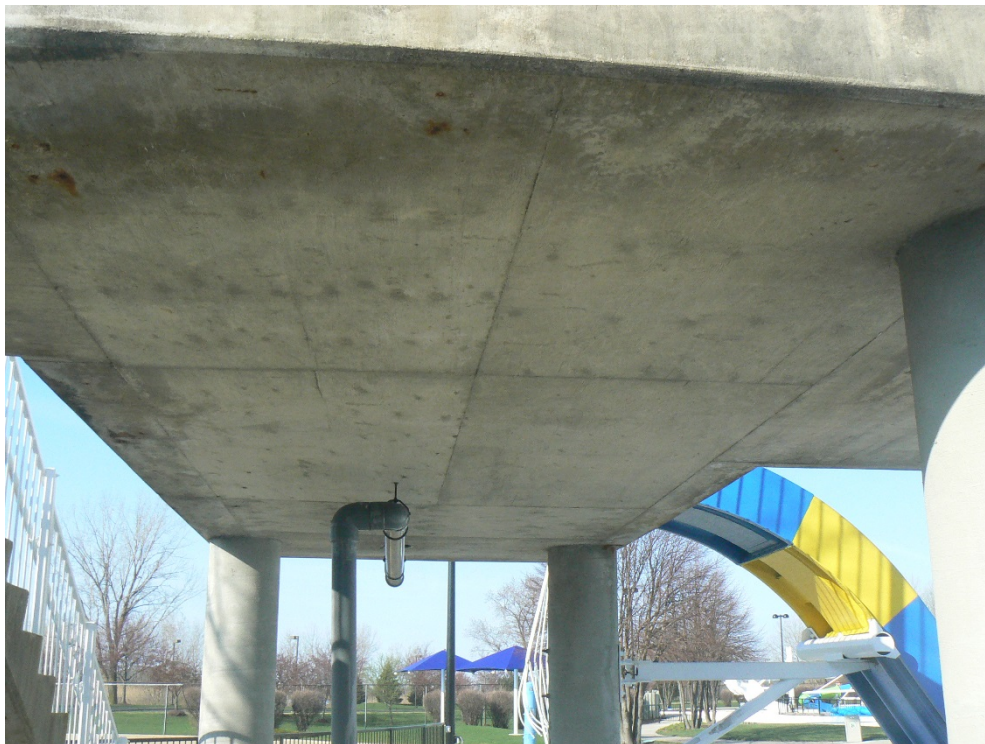
Underside of main platform
