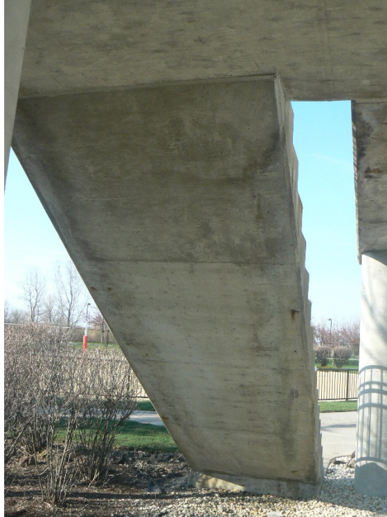
Underside of stairs
