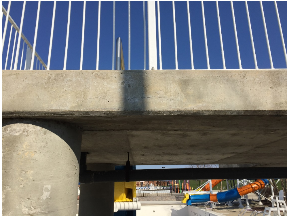
Side of main platform near southwest column
