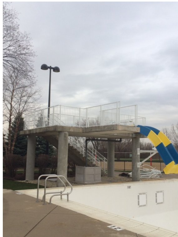
North Elevation of 3m Diving Platform
