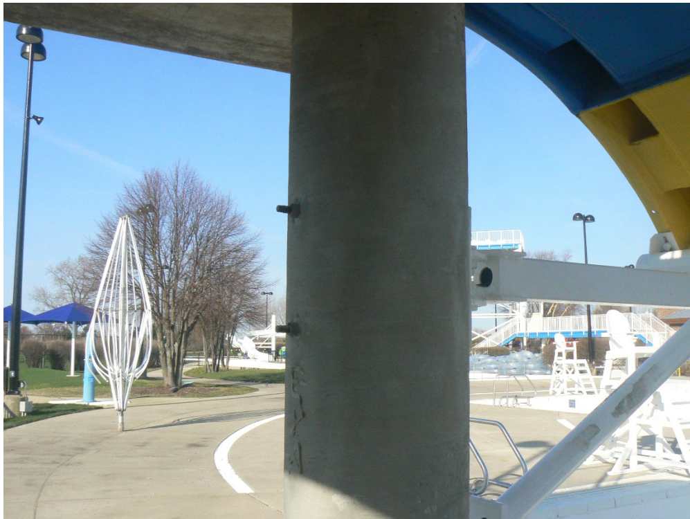
Slide attachment to northwest column
