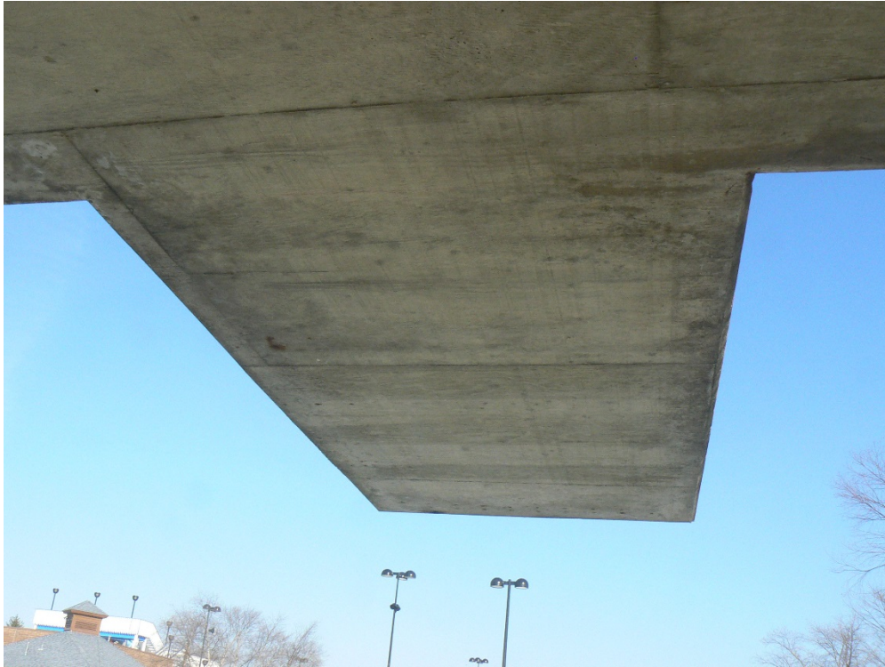
Underside of diving platform
