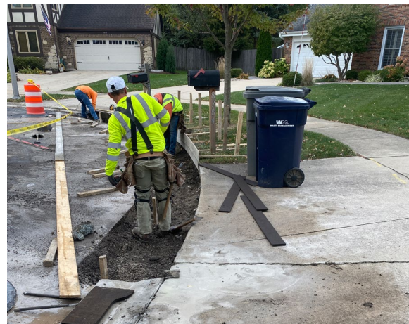
2020 Village Road Improvement Program
