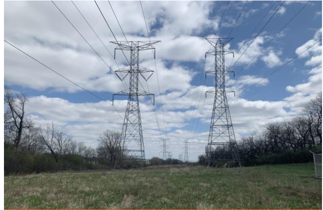
Commonwealth Edison right of way looking east at 110 th Avenue.
