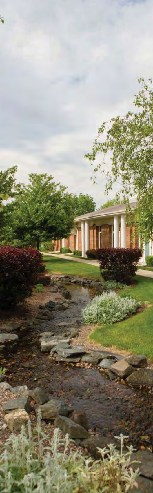
Ravinia Woods Office Center, Orland Park (Wehmeier, 2013)
