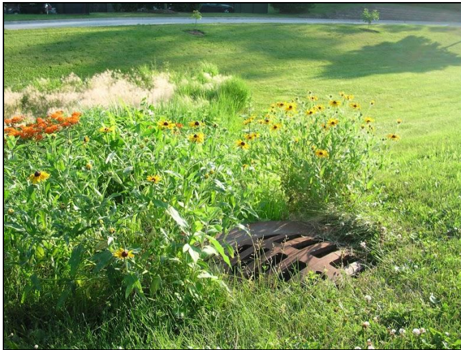
A pretty rain garden has been wisely planted near this storm sewer. The plants reduce the amount of water flowing into the sewer and clean out pollutants as the water runs through them. Photo courtesy of Jim Kleinwachter
