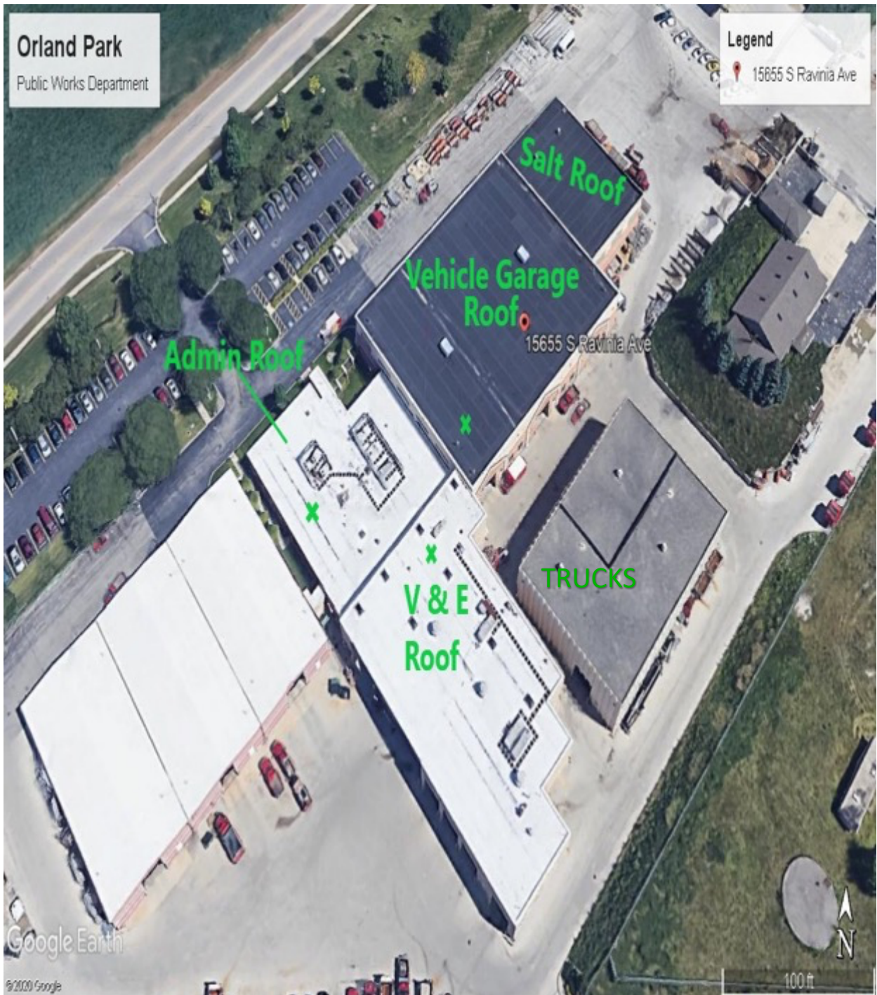
Green X indicates roof core locations
